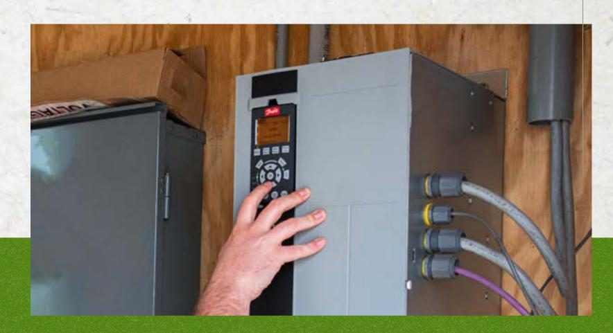
The VFD uses radio signal controls to tell our operators what's going on with each water well. Most importantly, its pressure sensors monitor water and energy usage, prevent erosion, and help us save on labor and fuel.
